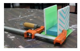
**Step 6:** Use a vice to pinch the tiles against the wooden block. Leave for 24 hours to let the glue bond completely.
